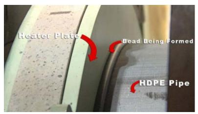
A good fusion process starts with the heat soak where the resin melt occurs slowly against the heater plate. Once the plate is removed, the bead is formed by the joined melted resin from both pipe ends. (Image: Alliance)
