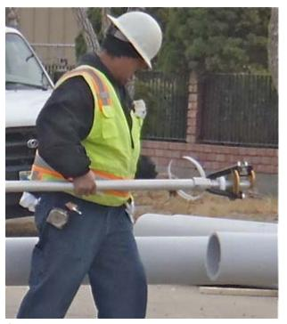
Several types of tools can be used to debead fused pipe. The one shown below is an internal debeading arm that can extend inside a pipe the full 50 feet if necessary. Note the operator is holding the cut, internal bead in his left hand. The pipe shown is grey, HDPE sanitary sewer pipe. (Image: Alliance)
