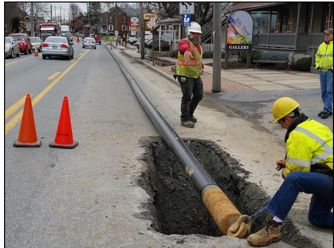
Replacing pipes with HDPE pipes in Pennsylvania Amish Country
