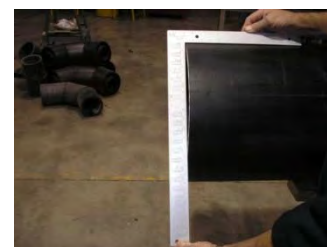
Figure IV-b - Measuring allowable gap with Carpenter's Square
