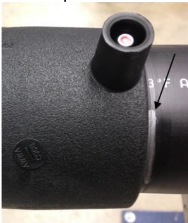
Stab depth is correct
