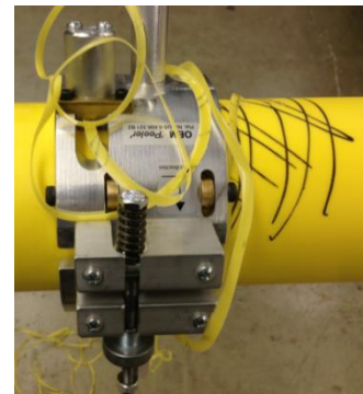
Figure X-e – Pipe Scrapping
