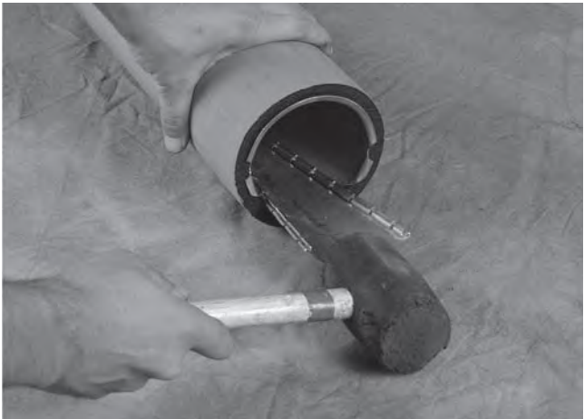
Figure 12 Install Split Ring Stiffener in PE Pipe
