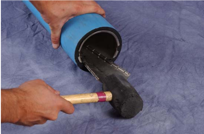
Figure 23 Install Split Ring Stiffener in HDPE pipe
