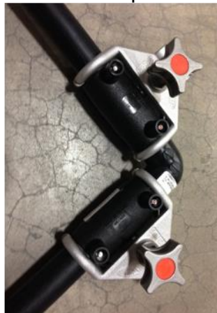
Alignment clamps used
