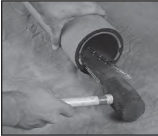
Figure 19 Install Split Ring Stiffener in PE pipe
