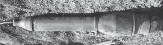
Figure 2 The Bursting Head of the Pneumatic System
