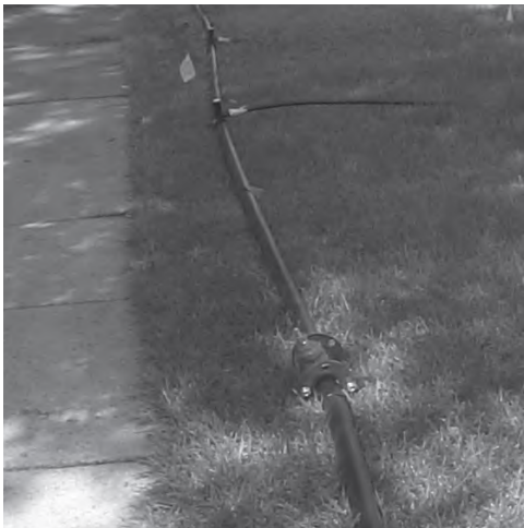
Figure 19 Example of Above Ground PE Bypass Pipe
